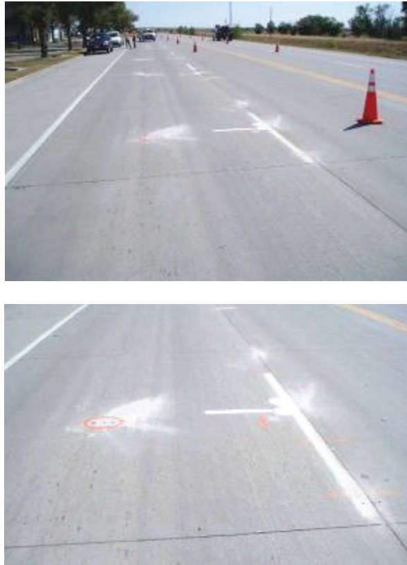
Figure 21. Overall view of the Hugo, Colorado, site and an image showing three temperature holes drilled in the center of the slab and paint marks along the longitudinal joint for FWD positioning.
